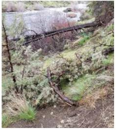
**TOP LEFT** The trail crew pulled limbs broken off the adjacent juniper trees and used them to block erosion gullies where water from the existing trail concentrates and causes problems. Side trails that access kayak access points and areas where fishermen access the stream were left open. Erosion gullies that lead to thick patches of willow brush that would prevent kayak or fishermen access were blocked to reduce the erosion impacts.
